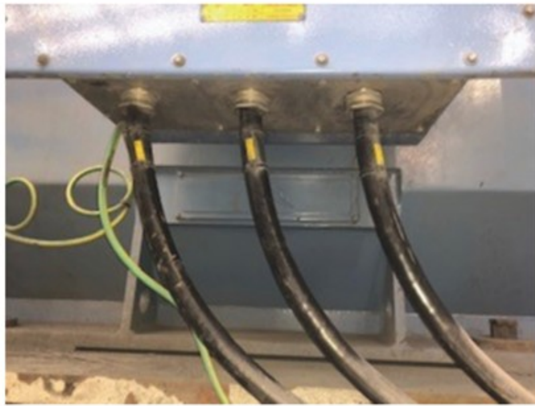
1. Lower front angle of incomer glands
